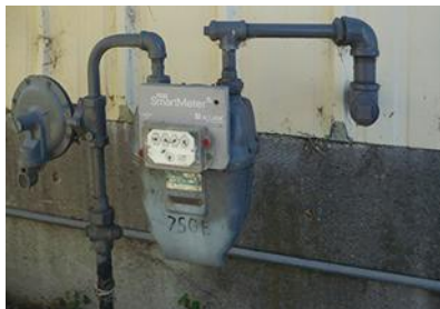
Smart meters, such as this one from Pacific Gas & Electric, have been one of the earliest applications for low-power wide-area networks. (Image courtesy of Ellin Beltz, via Wikimedia Commons)
